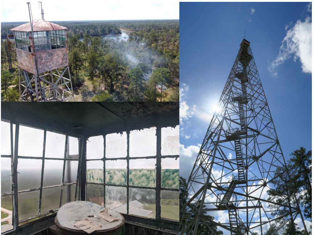
Mike Bell and Elliot Smith—The tallest fire tower in the northern hemisphere, the Woodworth tower in Alexander State Forest in Louisiana. At 175 feet tall, this Aermotor Model MC-39 is the second tallest in the world to a 200 foot tall tower in Australia—the Beard Tower.
