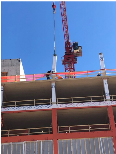
Once craned into position, final placement and attachment of this column took less than five minutes.
